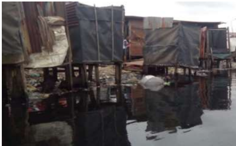
Plate 5. A typical toilet system in Makoko.
